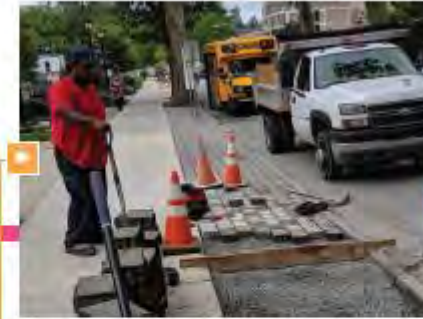
Installing permeable paving at West Chester University, West Chester Borough, PA.
