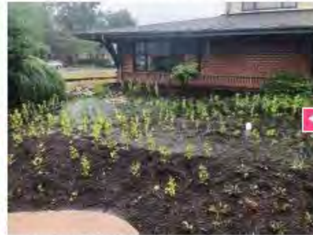
Newly planted rain garden collecting stormwater, West Grove Borough, PA.
