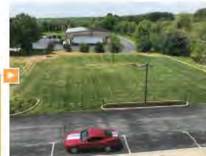
Pervious overflow grassed parking area at Dansko Company store and outlet, Penn Township, PA.
