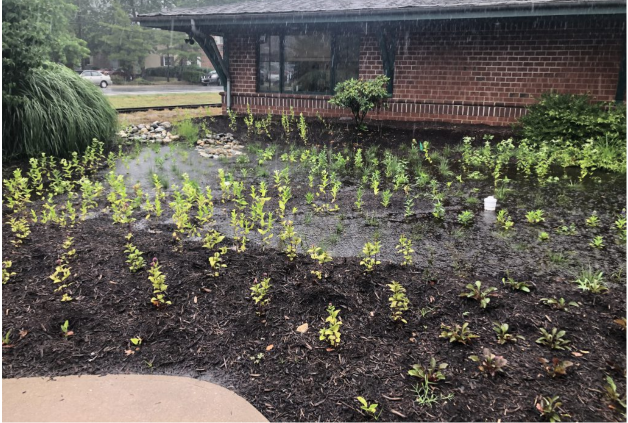
Recently installed rain garden full of stormwater during a two-inch rain storm in July 2020.
